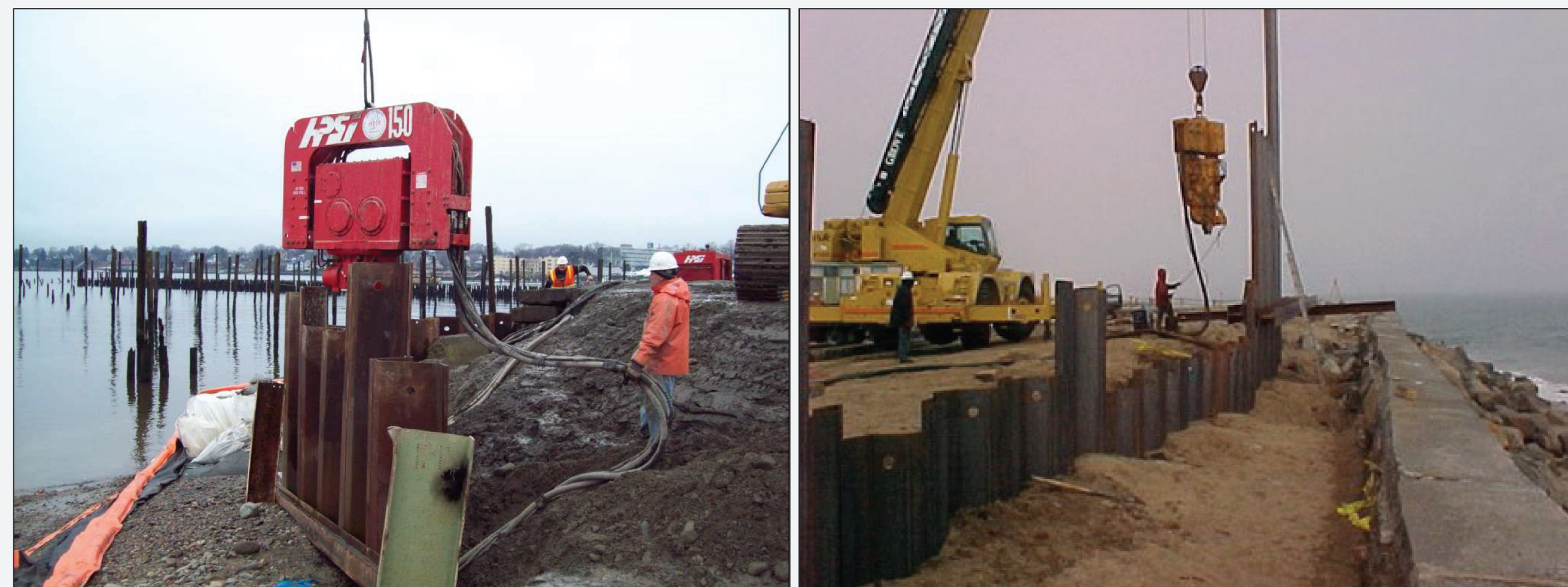
Construction of Barrier Wall - Sheet Pile Installation
