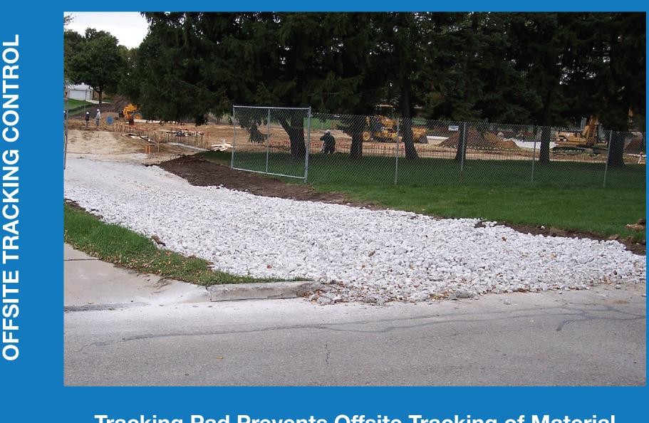
Tracking Pad Prevents Offsite Tracking of Material
