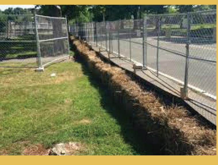
Silt Fencing with Hay Bales Limits Erosion
