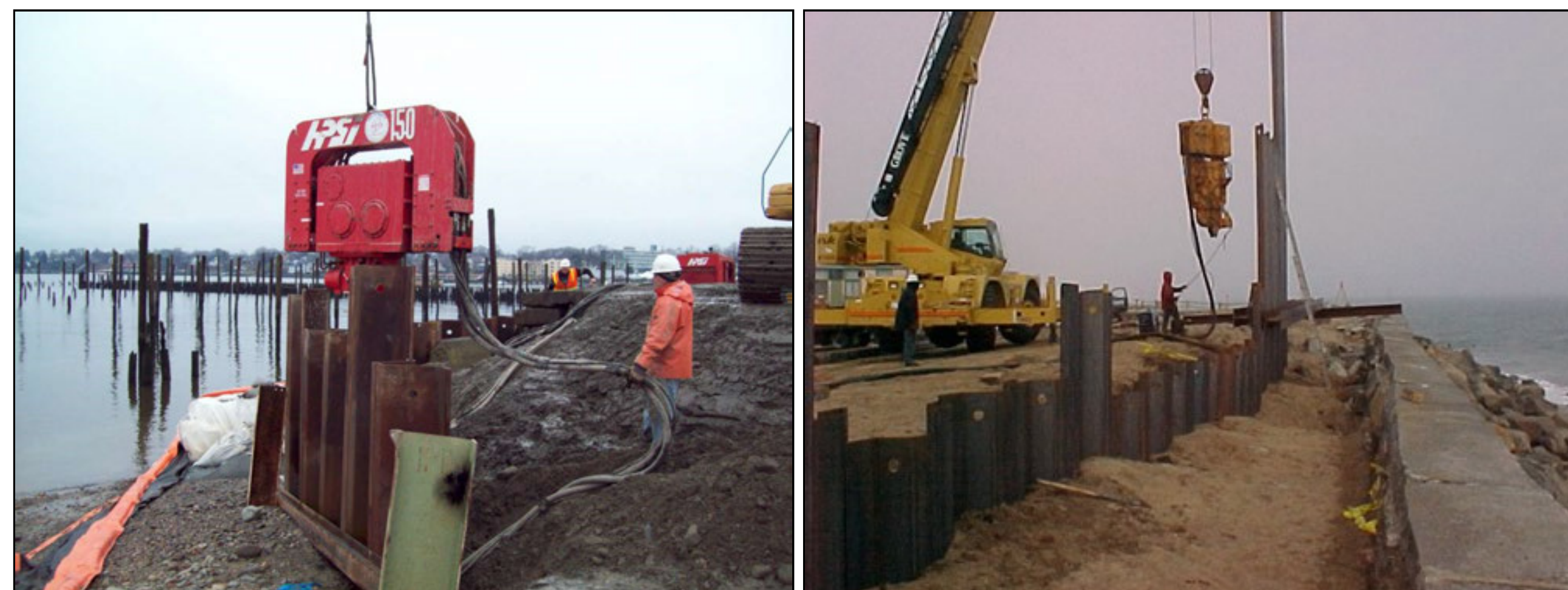
Construction of Barrier Wall - Sheet Pile Installation
