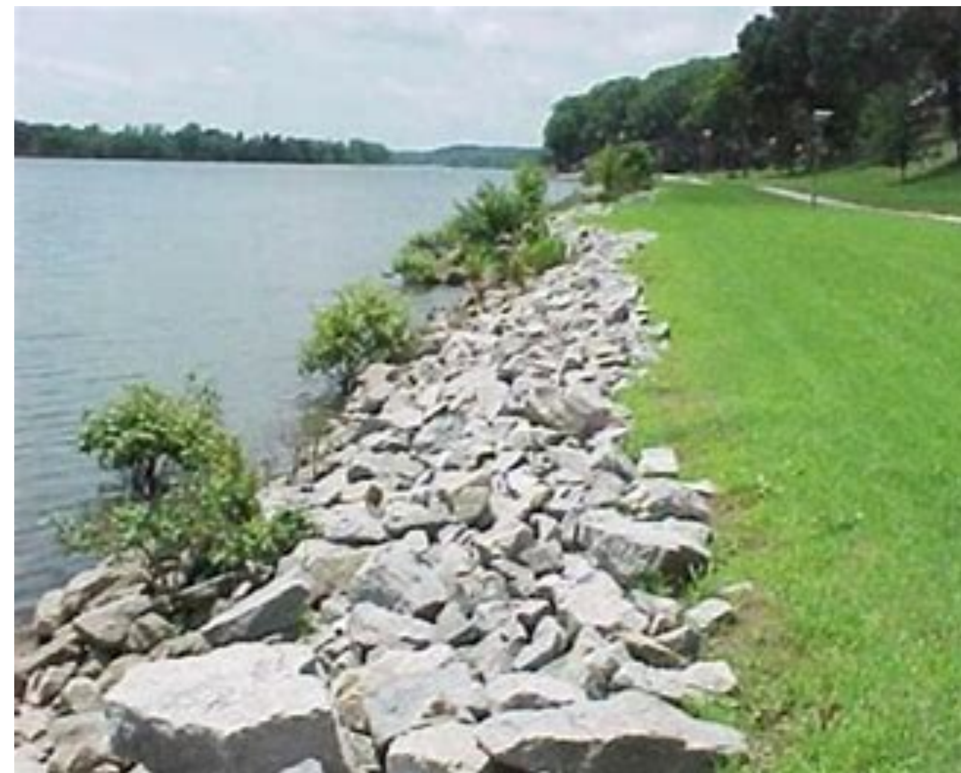
Example of a Riprap Revetment
