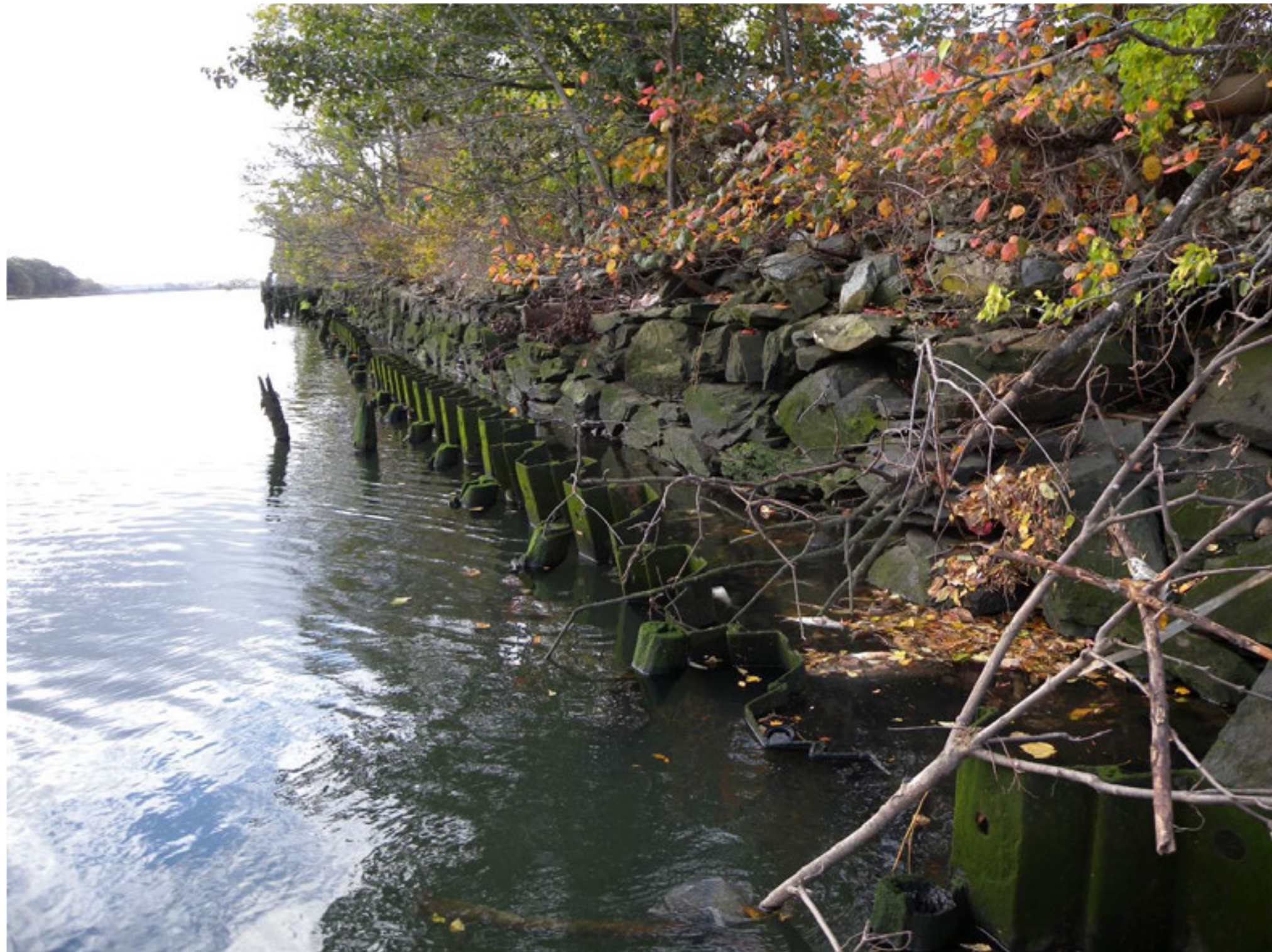
Granite Stone Block Wall and Steel Sheeting
