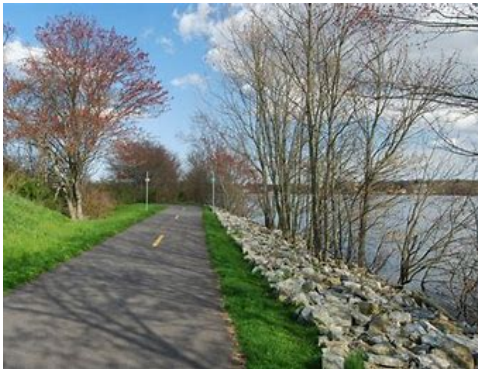
Example of Bike Path with Adjacent Revetment
