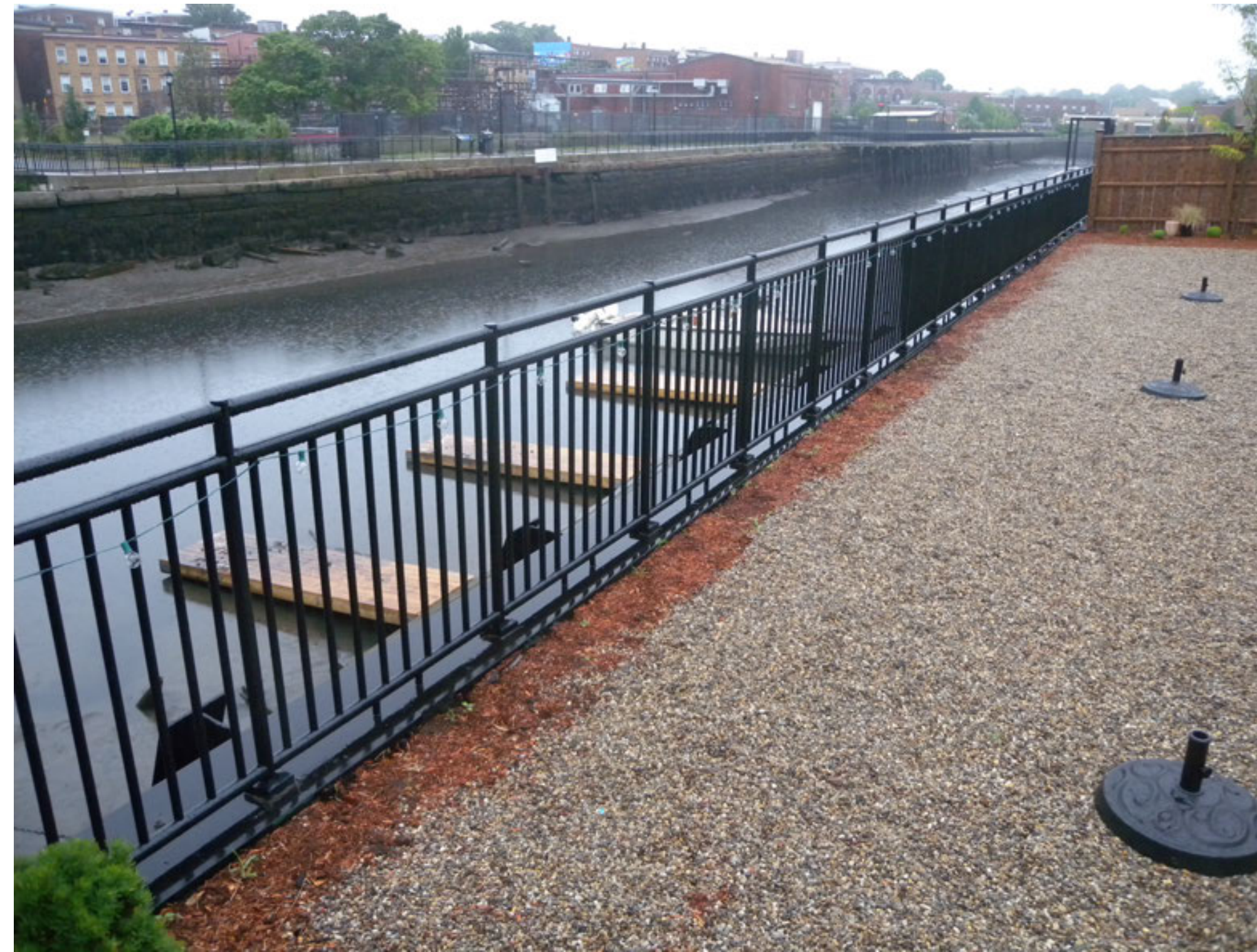
Example of Bulkhead Railing System
