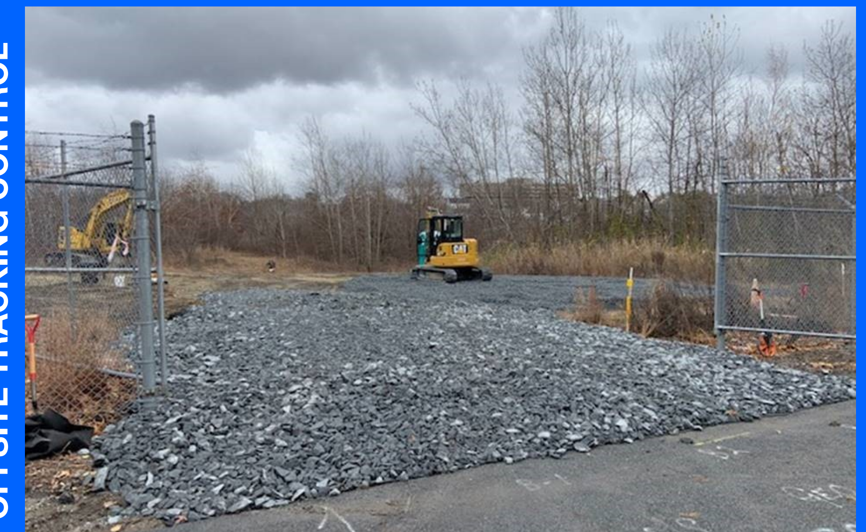
Tracking Pad Prevents Offsite Tracking of Material
