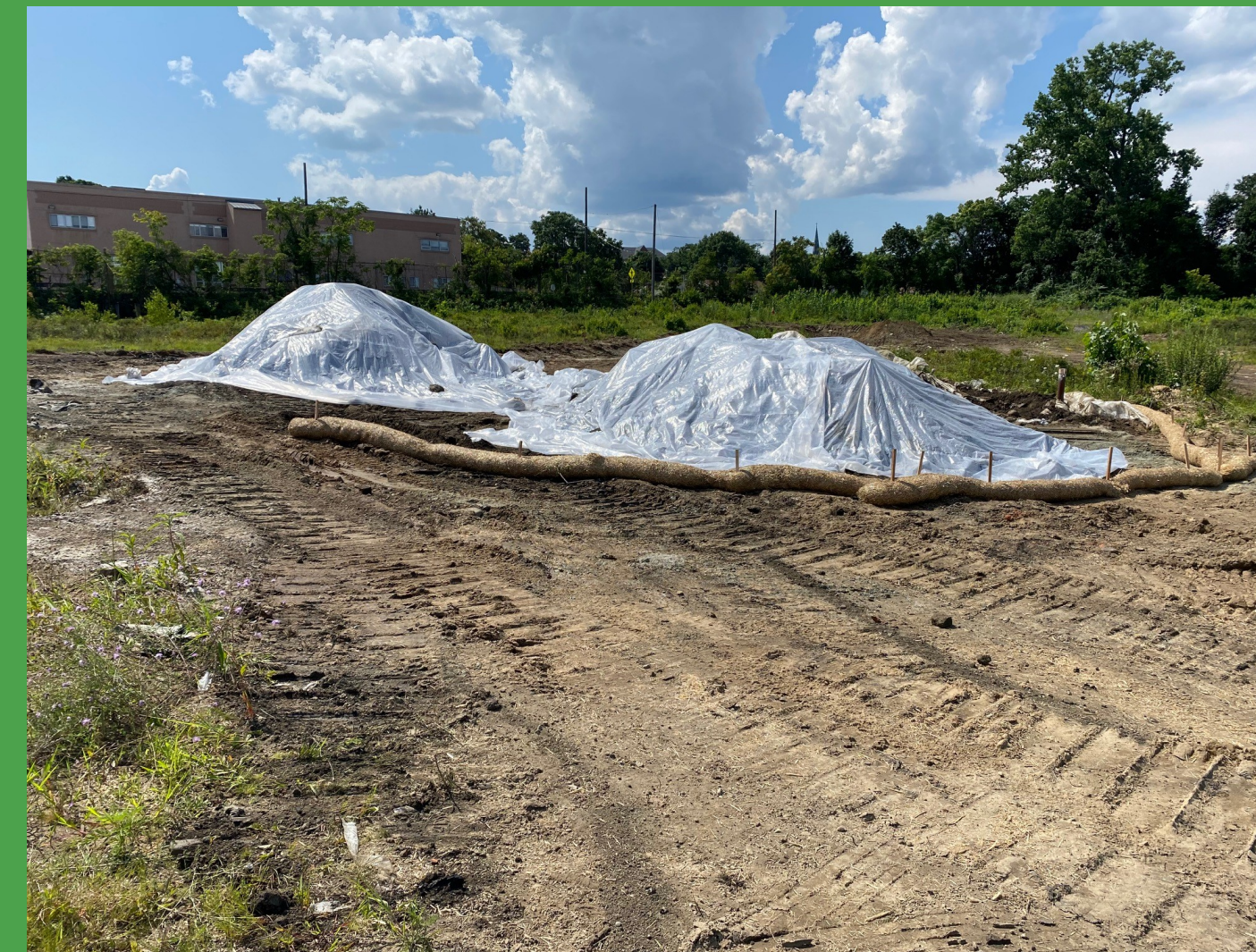
Covered Stockpiles Control Dust and Odors
